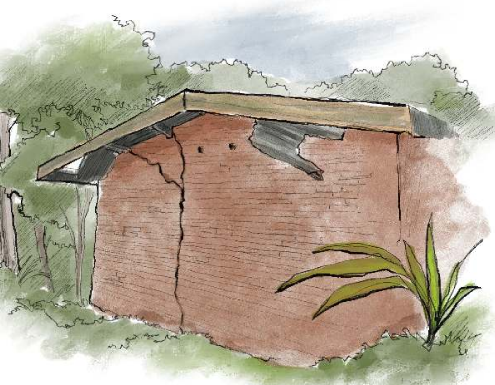
Illustration 21 : The wall of a resident's house near the mining area had a heavy crack.
