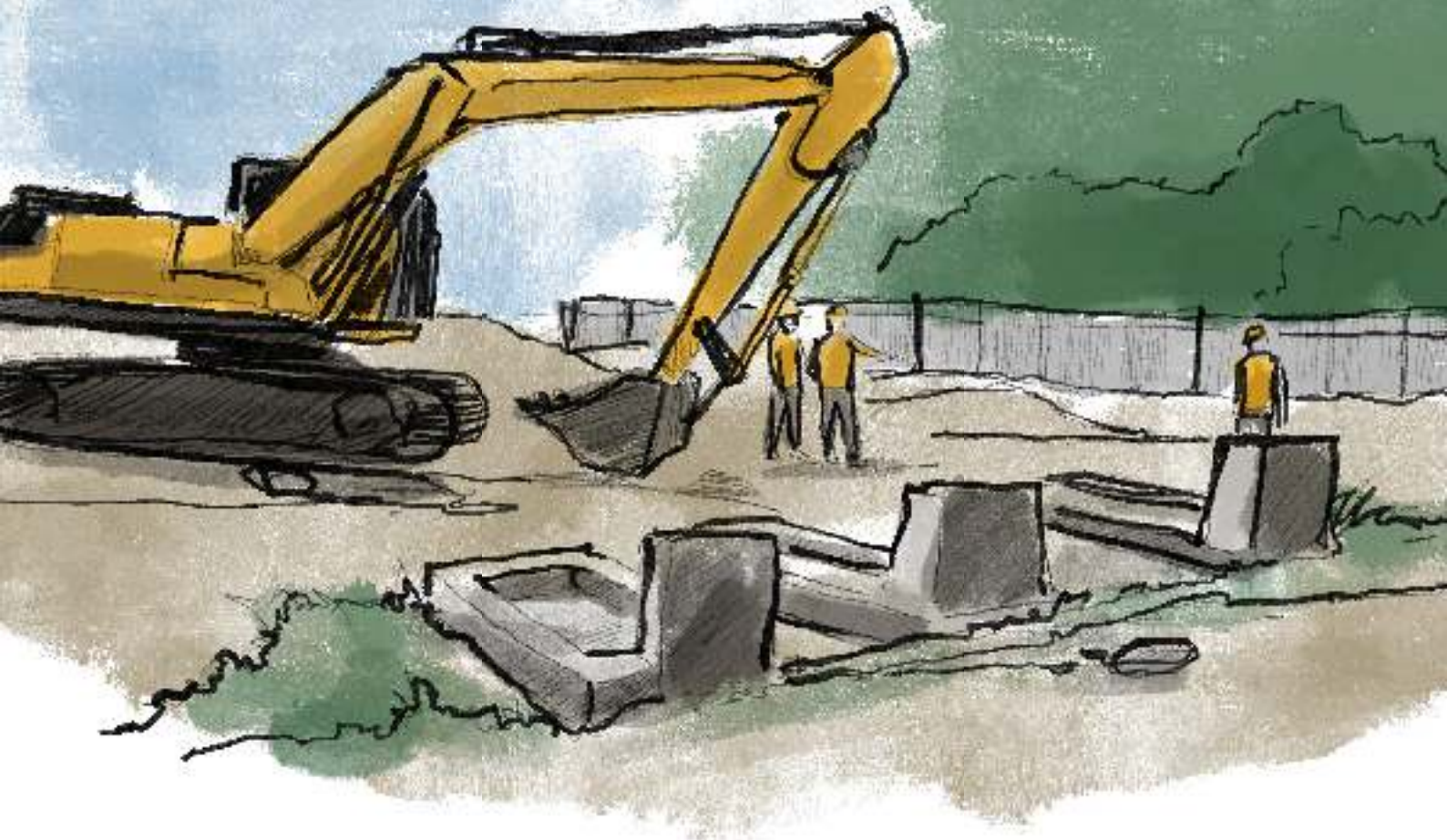
Illustration 9: The company excavated and widened an existing road.
